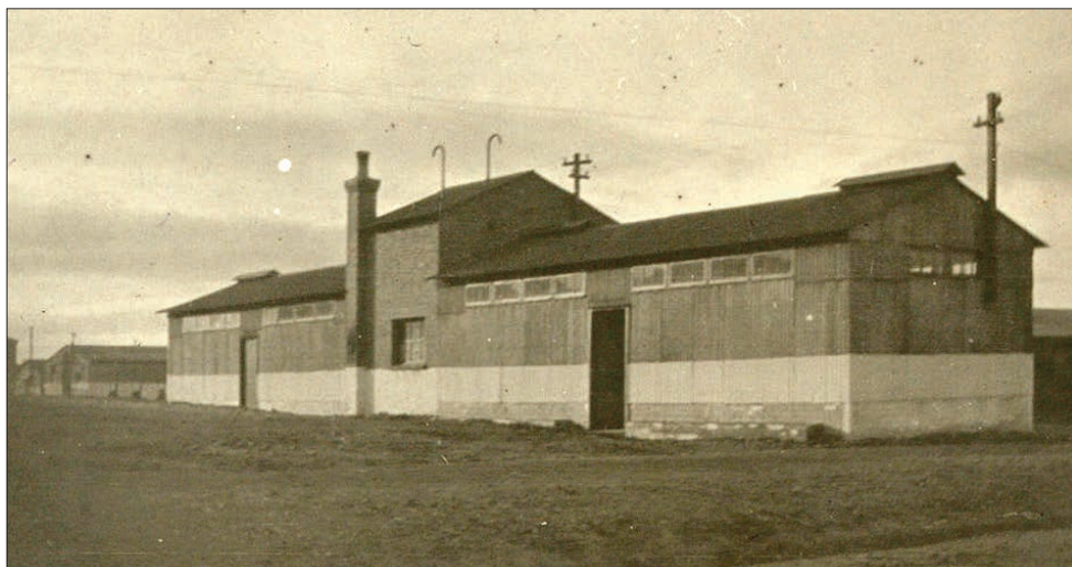
Top, The bathhouse foundations and above, a WW1 photograph of a bathhouse.
